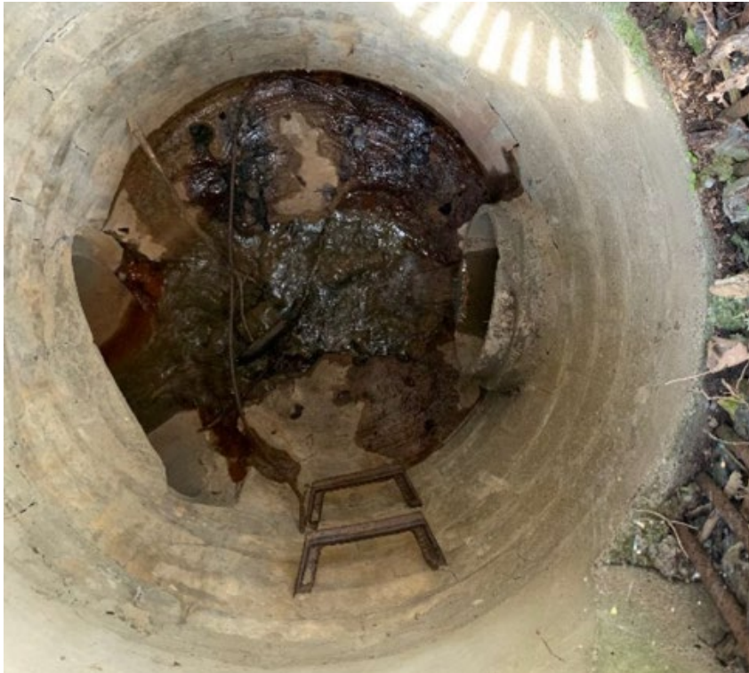
Downstream End of Pipe
