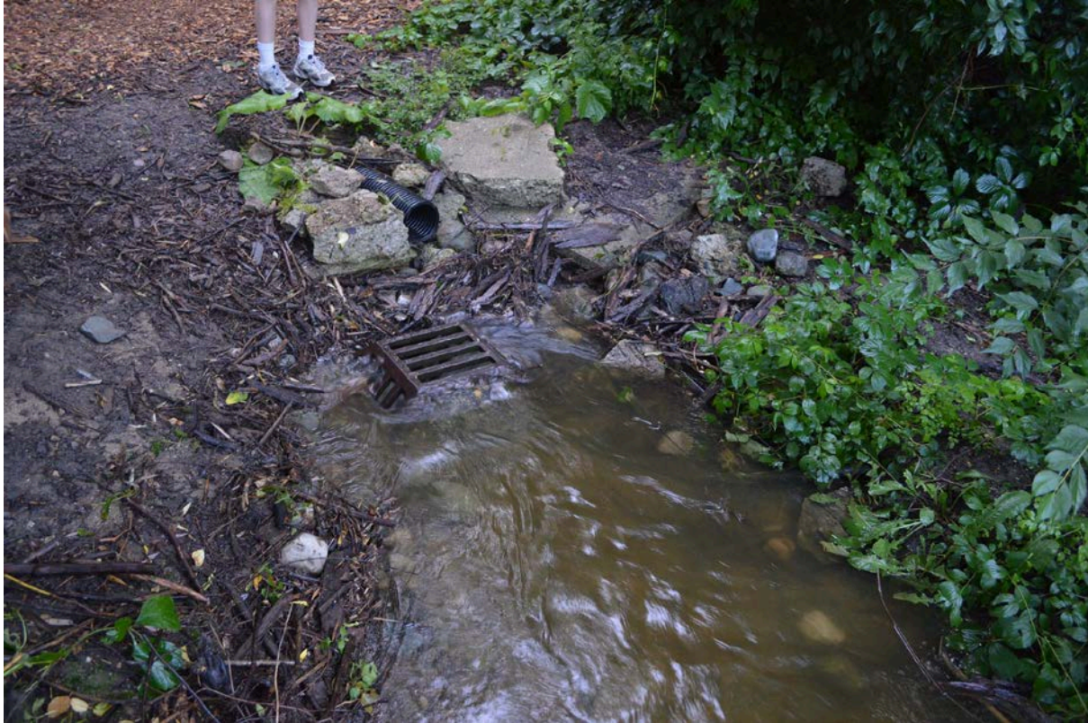
Figure 6: Existing Thurston Pond outlet at the beehive grate.
